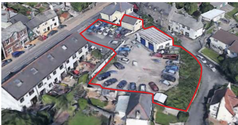
Env9: Land at South Devon Repair Garage
